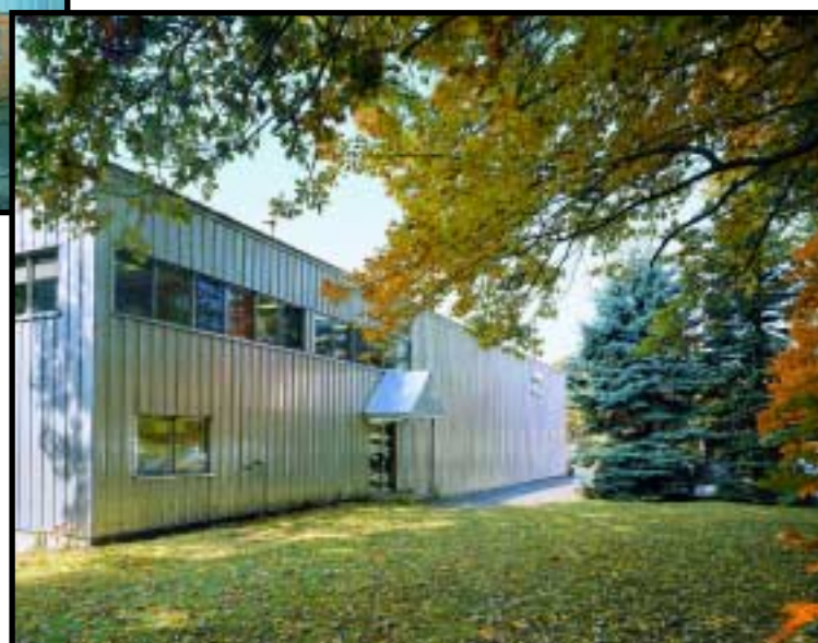
Standard and custom power units are assembled in Ashland, Massachusetts. This facility, 25 miles (40 km) west of Boston, also is a warehouse serving North American distributors.
